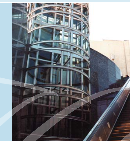
Sunset/Vermont Red Line Station
