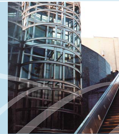
Sunset/Vermont Red Line Station
